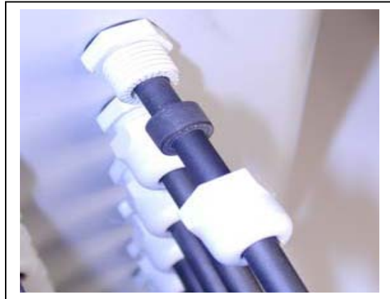
Figure 11. Connecting Cables to Enclosure
